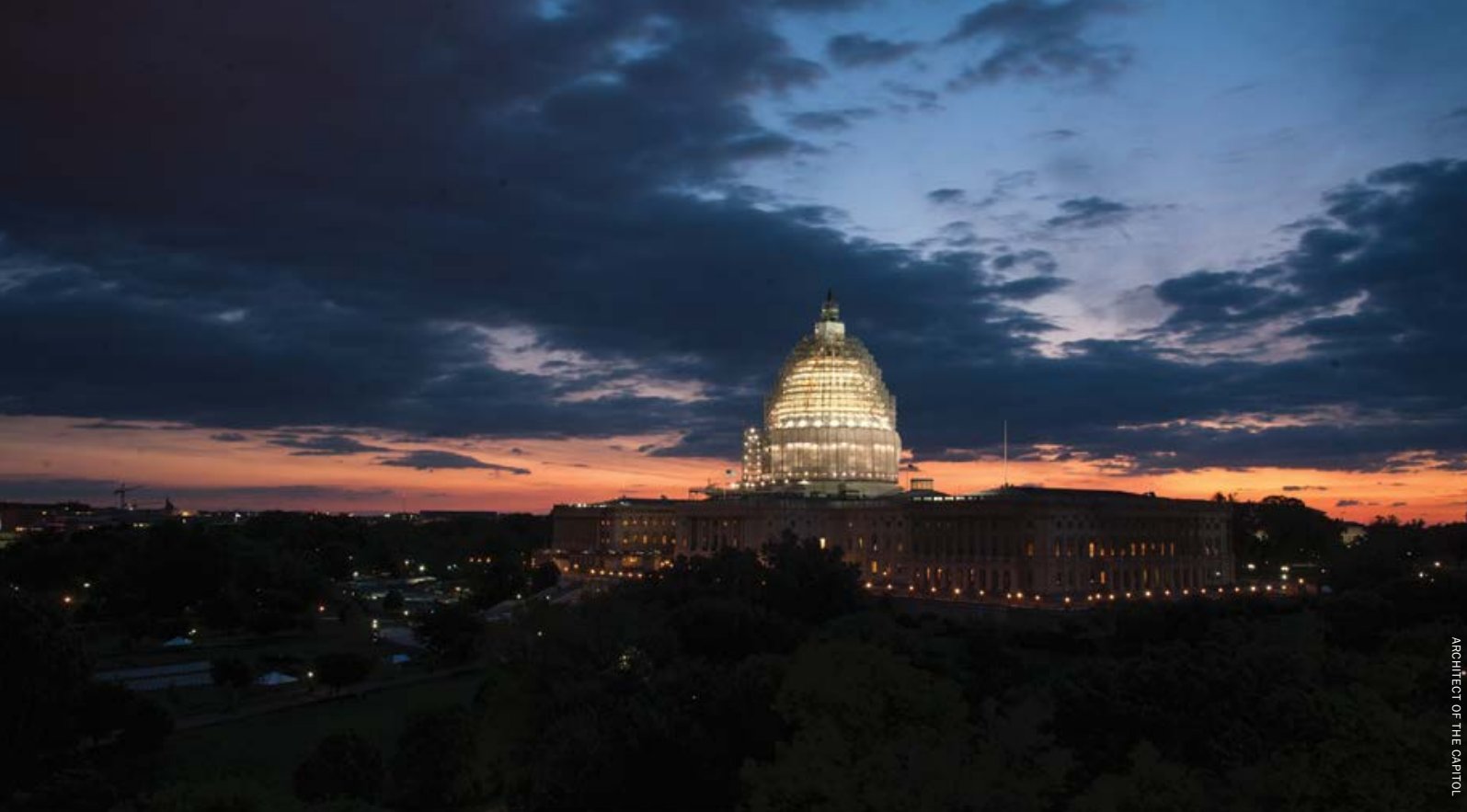
The Architect of the Capitol has begun the final phase of the Dome Restoration Project.
